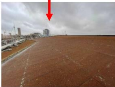
Sloped bitumen covered membrane over the RAAC plank roof
